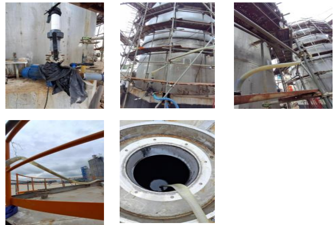
Fig. 2. Actual piping installation in hydrotest system
