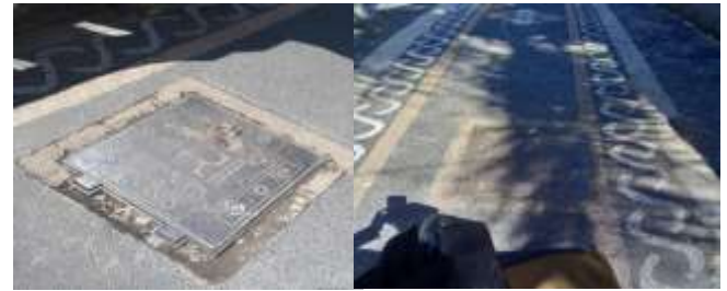
Figure 7. The Condition of Waterwaste Management in Pancor Village
