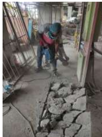
Fig. 3. Crushed Demolished Concrete
