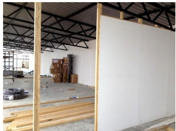
Enviroboard Installation Source: georgehill-timber.co.uk
