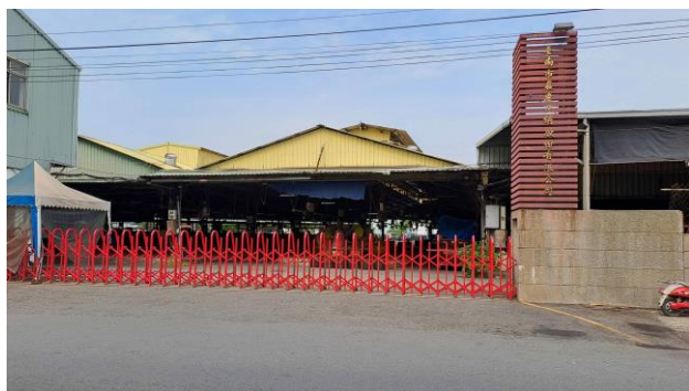
Fig. 3. The former site of the cattle market [8].
