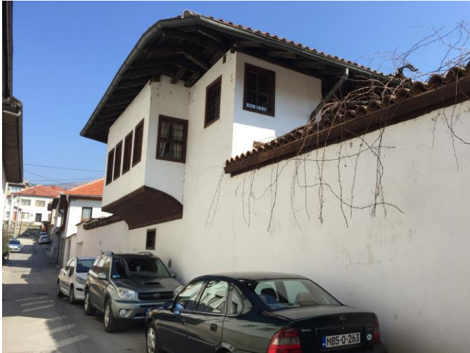
Figure 16. The Svanzo's house. Doksat towards Glodjina street Source: Author (12.19.2015.)
