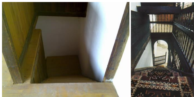
Figure 17. Wooden staircase (basamac) in Sabura's house (left) and in Svanzo's house (right) Source: Author (12.19.2015.)
