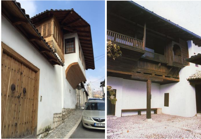
Djerzelez's house (left) and Svrzo's house (right) Figure 13. Vertical plan of an oriental-type city house in Sarajevo Source: Author (3.19.2016.)
