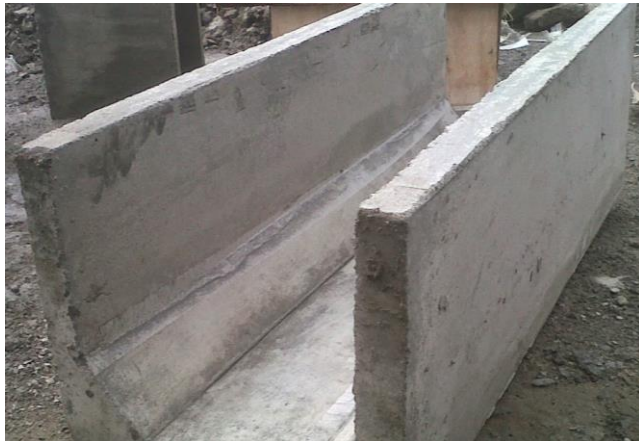
Fig. 4. The result of low-strength concrete production with the addition of Lusi material
