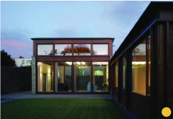
Fig. 31. Outside Office Entry
