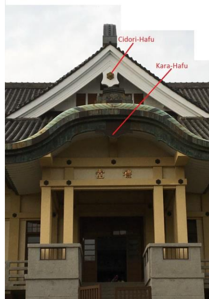
Fig. 2. The temple architectural form of Irumaya-zukuri is the most important formal feature of Bu-do-ku-den.
