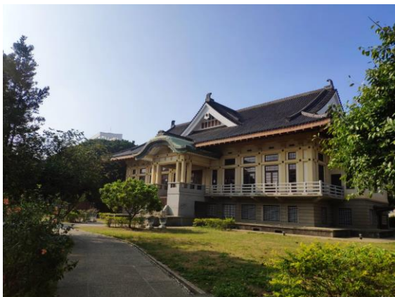
Fig. 3. A hybrid style of Japanese-Western Eclectic Architecture with faux column and beam frame walls.
