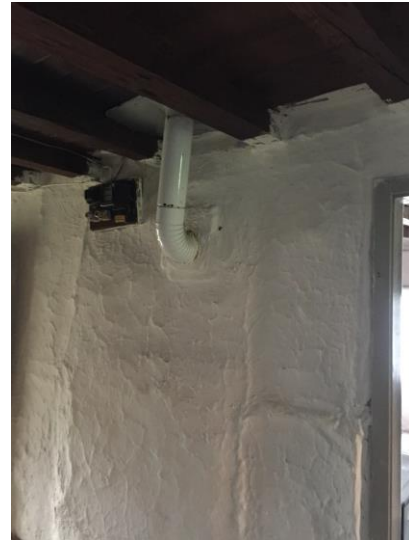
Figure 34. The flue from the furnace in the loggia first passes into the space of the hayat, and then through the poison into the space of the attic Source: Author (7/27/2016)
