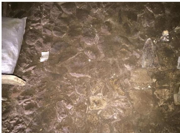
Figure 21. The floor covering on the ground floor is an extremely high quality cobblestone Source: Author (7/27/2016)
