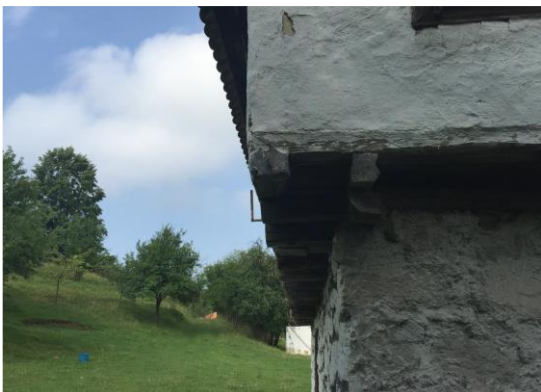
Figure 14. Cantilever overhang of the floor into the space outside the contour of the ground floor Source: Author (7/27/2016)
