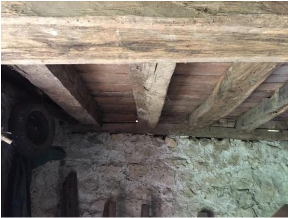
Figure 16. Wall surface and ceiling on the ground floor Source: Author (7/27/2016)
