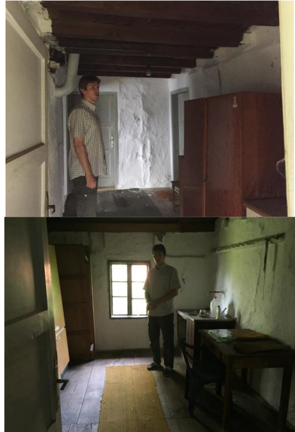
Figure 10. The space of the former “kuća” on the first floor. At the place in the outer wall, where the window is now, there used to be a door to the annex area where there was a “vodnica” and a toilet
