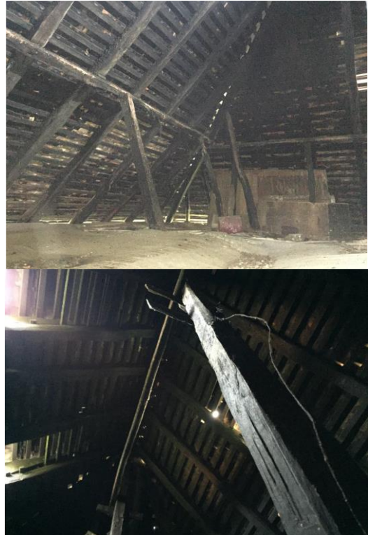
Figure 15. Roof construction (left). Part of the roof structure (upright chair with wooden bar for drying meat (right) Source: Author (7/27/2016)
