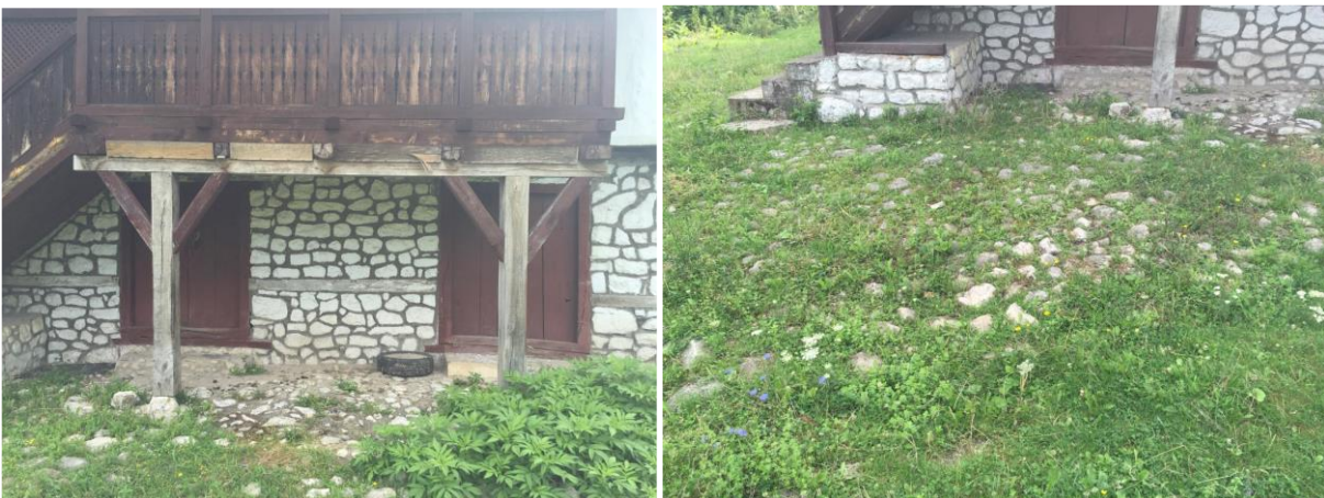
Figure 6. Porch at the entrance to the ground floor, below the sofa on the first floor (left). Due to the (once) intensive traffic of people, goods and livestock, the floor covering of the courtyard is made of stone cobblestones (right) Source: Author (7/27/2016)
