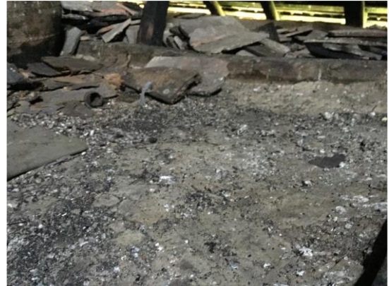
Figure 24. Floor in the attic Source: Author (7/27/2016)
