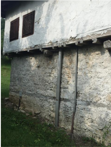
Figure 7. At the place where there used to be an annex with a “vodnica” and toilets, water was brought and a sewer drain was arranged from the newly renovated sanitary facility in a large chardak, along the wall of the former “kuća”.
