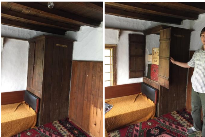
Figure 33. Bathroom in the form of a closet in one of the balconies. This bathroom has a bathtub as Figure 32. Source: Author (7/27/2016)
