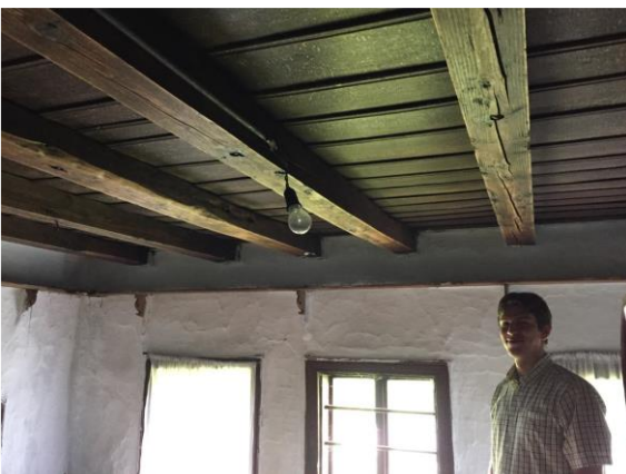
Figure 18. White painted wall surfaces and patinated wooden ceiling in one of the chardaks. The boards are made of beech wood Source: Author (7/27/2016)
