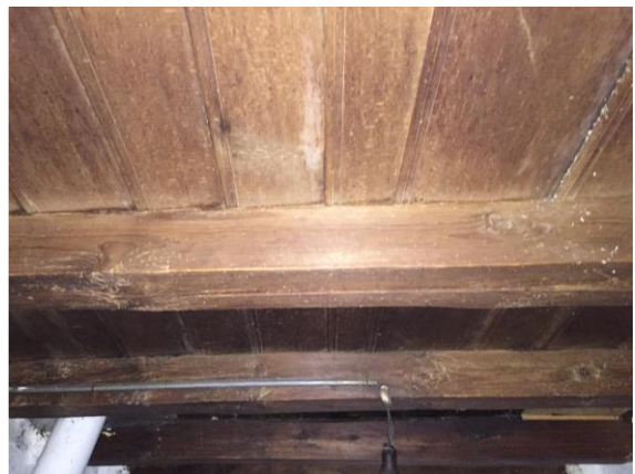
Figure 20. Wooden ceiling attic in the space of the hayat Source: Author (7/27/2016)
