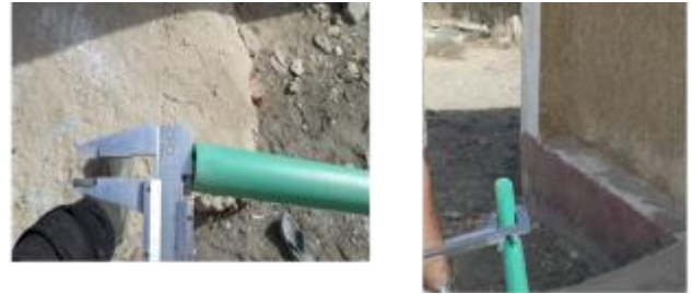
Figure 13: Quality control for pipelines
