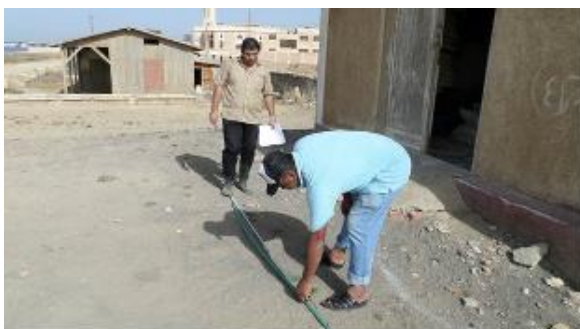
Figure 12: Quality control for pipelines
