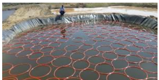
Figure 27: Implemented master solar pond
