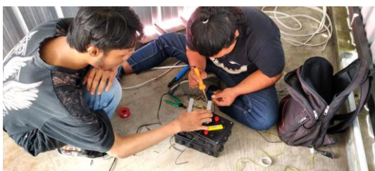
Fig. 2. Installation a datalogger and test a serial communication.
