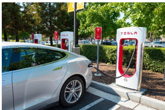
Fig. 6. Tesla's Charging Station which is spread across America can charge Tesla cars for free because it gets a free supply of electrical energy from the sun by utilizing solar panel technology [10]
