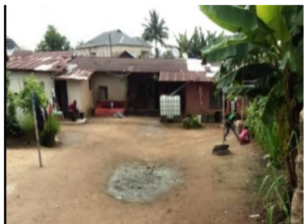
Plate 2 and 3: Fabricated Buildings with rooms facing each other
