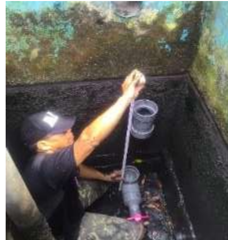
Fig. 15. The installation of filter
