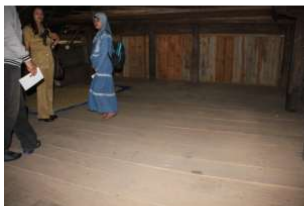
Figures 4. Condition of Toba Batak traditional house space in the middle and back that does not use partitions
