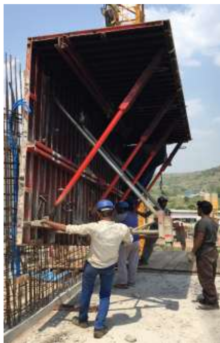
Fig. 4. Placing the Tunnel formwork with the help of tower crane.
