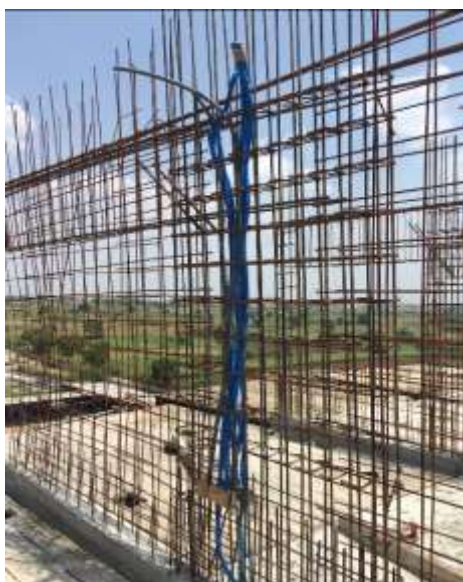
Fig. 3. Reinforcement and conduit work for wall Slab.
