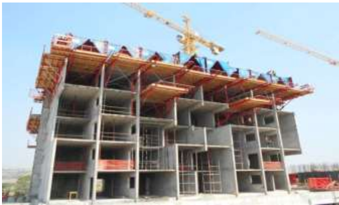
Fig. 6. F2 Building during tunnel casting.
