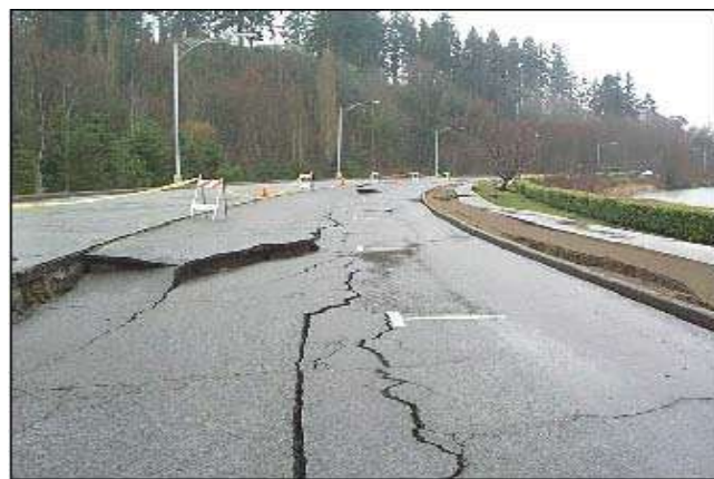
Fig. 4. Example photo documenting site damage, imaged along North Deschutes Parkway showing a lateral spread toward Capitol Lake, which is to the right of the photograph. All photos were georeferenced and dated (from Bray, et al, 2001).
